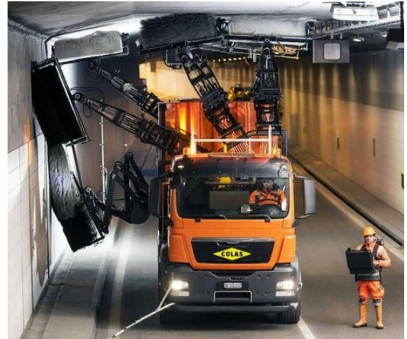
Figure 10. Tunnel cleaning system [55]
