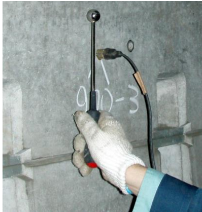
Figure 3. Inspection using an impact hammer [17]
