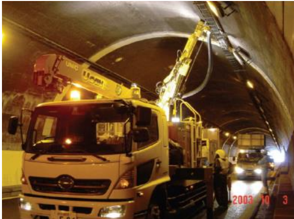
Figure 8. Void detection rotary percussive drilling machine [52]
