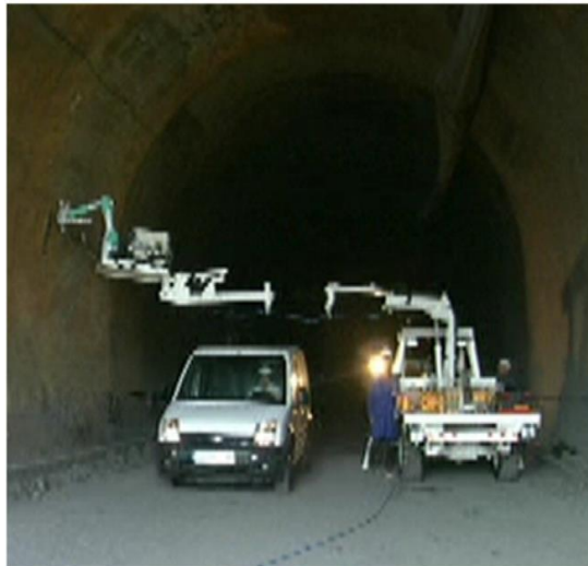
Figure 18. TunConstruct system test in a Spanish tunnel. Note that one lane of the tunnel traffic flow is not blocked
