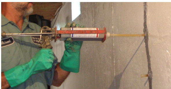
Figure 1: Conventional manual procedure of fissure injection
